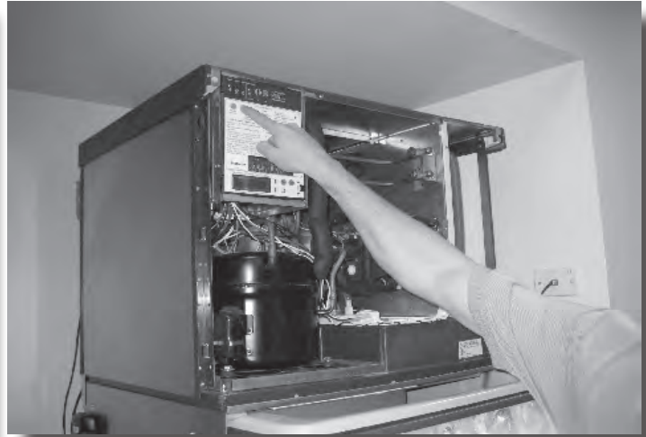
15. Re-assemble all and push Clean button.
